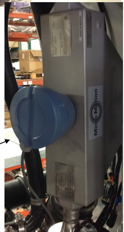
The products flow through the mass meter flowmeter.
