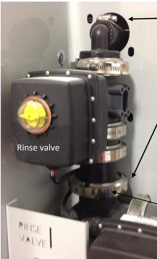
Remove these two clamps to remove the rinse valve assembly. The rinse valve assembly will go inside the cabinet after valves 5 & 6 are attached.
